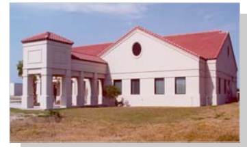
Patrick Air Force Base Medical Training Facility
